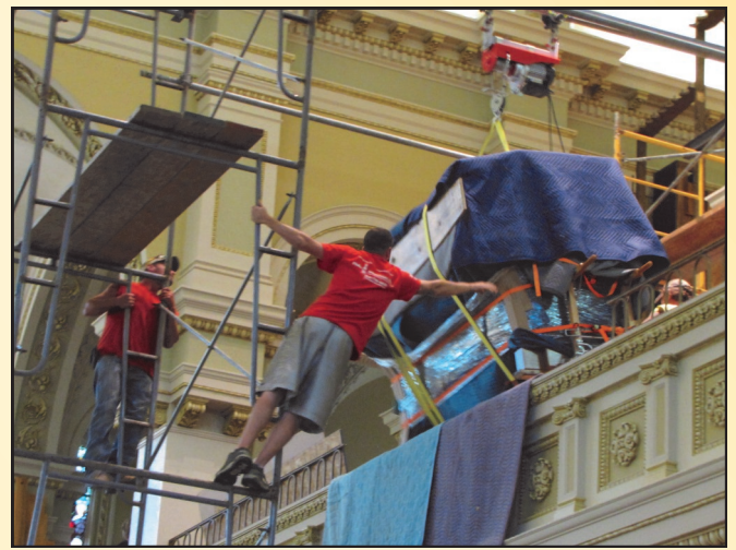
~Lifting the organ console up to the organ loft~
