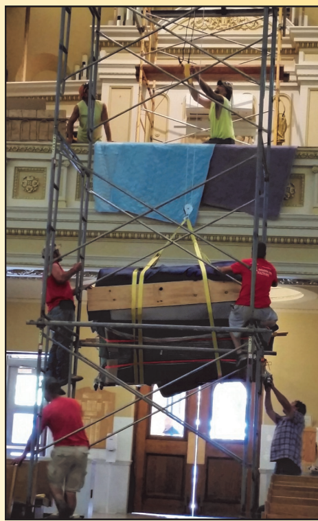
~Lifting the organ console up to the organ loft~
