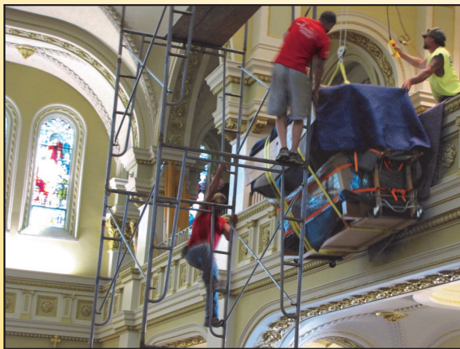
~Lifting the organ console up to the organ loft~
